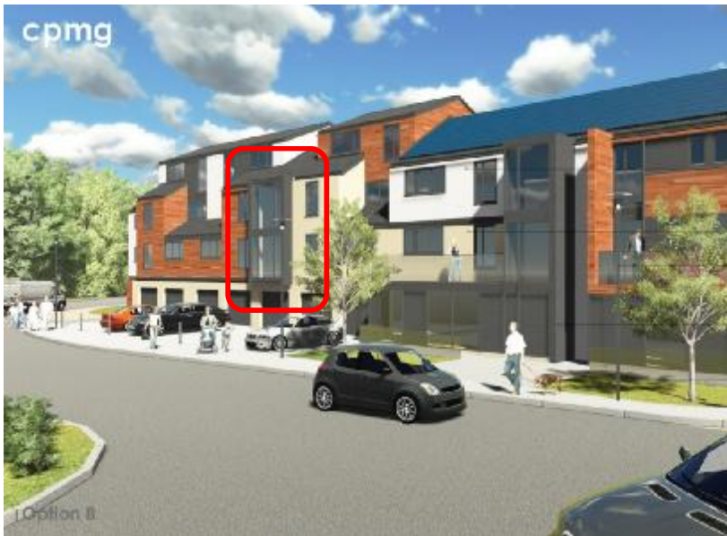
Cantilever balcony extensions (as highlighted)
