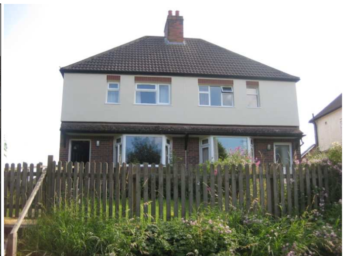
Figure 5: After External Wall Insulation
