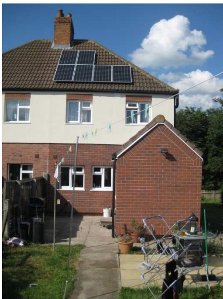
Figure 6: With 6 Solar Panels
