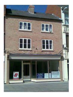
The former P & M Fruit Shop on Nottingham Street has benefited from a completely new shop frontage, the former aluminium folding doors replaced by traditional timber elements, with off centre recessed door and new tiled threshold. The green paint was removed from the upper storey brickwork and new timber windows with stone cills inserted. The roof was re-slated and the chimney stack and pots restored.
