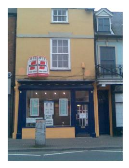
No 16 Market Place is currently occupied by Herbal Health. The building has been totally restored with the concrete pre cast tiled roof replaced in natural slate and the chimney stacks and pots refurbished. The inappropriate plastic internally illuminated box fascia sign has been removed and the shop front, one of the most traditional within the town centre repaired and redecorated. Missing elements from the top of the fascia board have been replaced and releaded.
